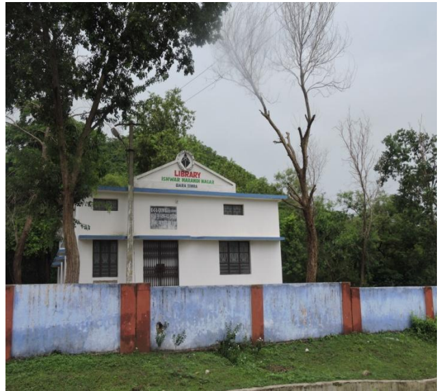
Plate -12: Library constructed under CSR activities at Ishwar Marandi Nagar, Bara Simra
