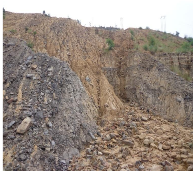
Plate -4: Severely eroded with deep rills and gullies on the slope of the inactive back filled OB dump area
